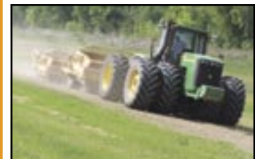
Filling erosions and washes.
