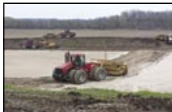
Covering sand berm.
