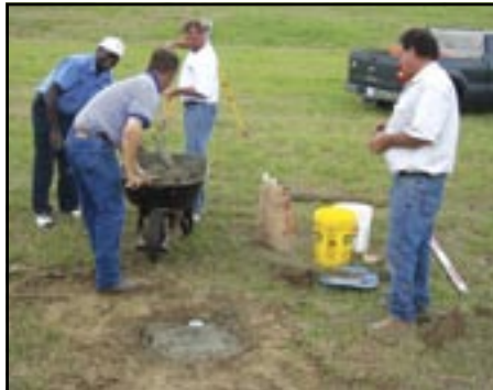
Crew setting benchmark in concrete.
