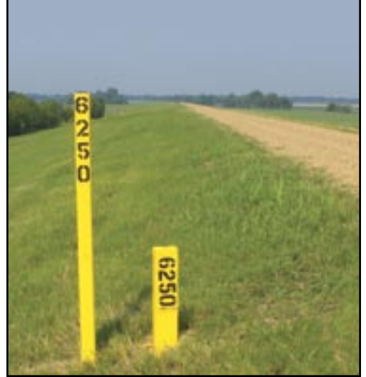
Completed station marker.
