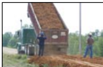
Graveling top of levee.
