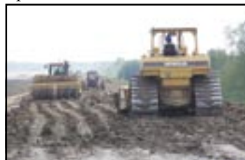
Topping out the levee.
