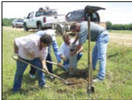
Crew setting station marker.
